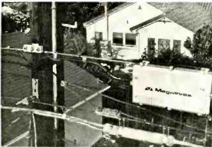
IDEM, NERVE CENTER OF THE SYSTEM, is the liaison between subscriber and head end.
